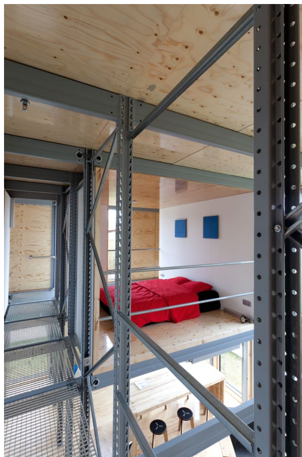
Inrichting Nul-energie woning Team Belgium: Ghent University
